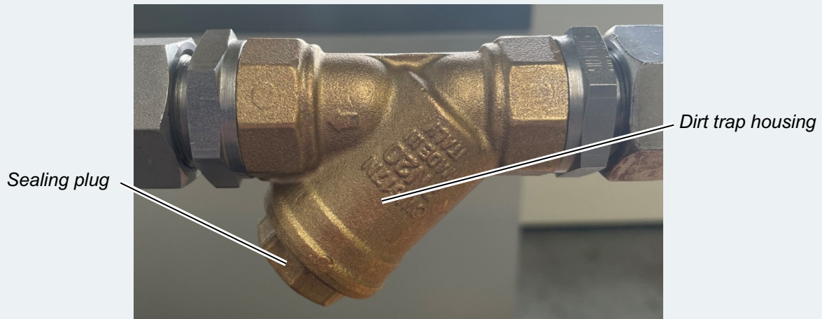
Figure 4: Dirt trap housing
